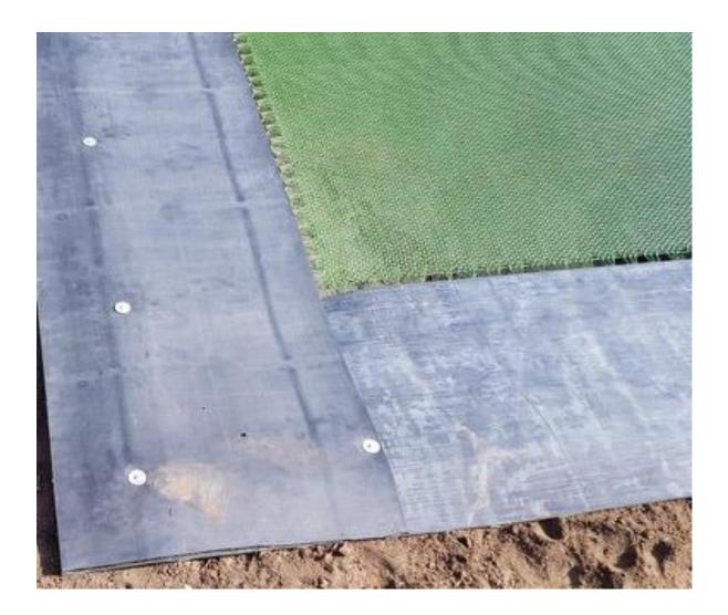
**Step 5:** If there is excess rubber across either of the ends, you can use a metal ruler with a Stanley knife to carefully trim back the rubber.
