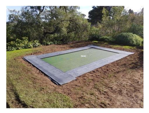
**Step 4:** This stage you will need a **hi-impact drill or ratchet gun with a Phillips head drill bit.** Place your screws and washers around the rubber, **Note:** 3 Screws and washers should be placed in each corner and then a washer spaced every 300-400mm apart.
